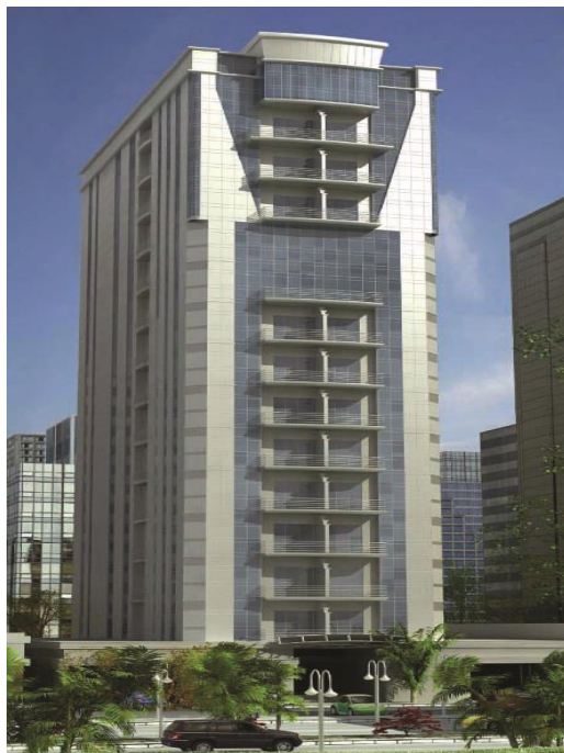
ELECTRICAL WORKS @ 2B+G+14+GYM BUILDING @ AL BARSHA FIRST
