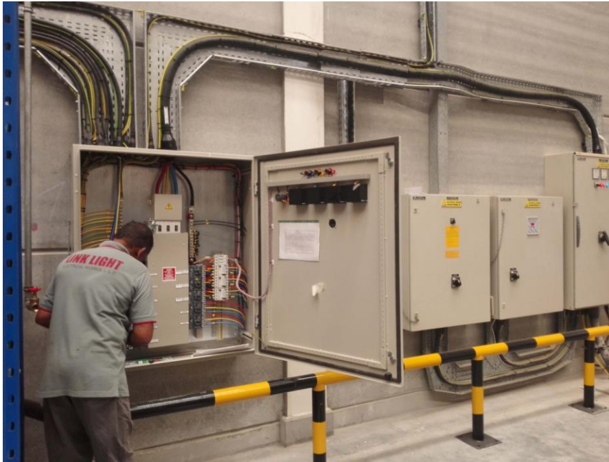
ELECTRICAL WORKS @ METALOCK INSITU MACHINING MIDDLE EAST LLC, DUBAI MARITIME CITY
