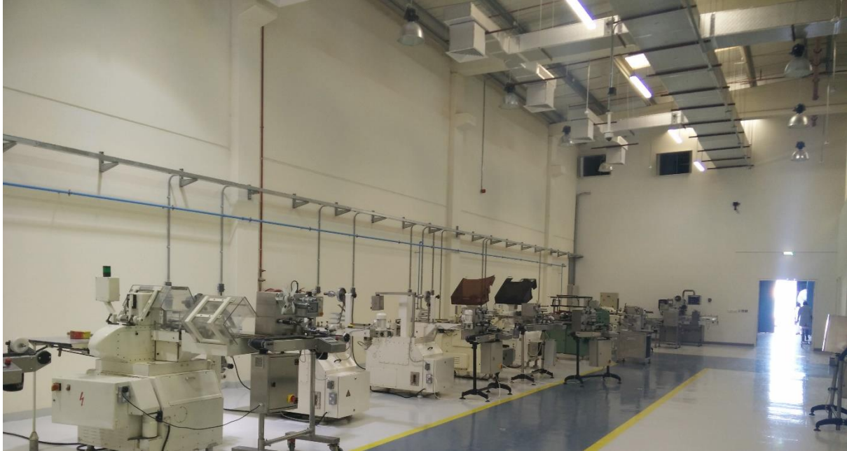
ELECTRICAL WORKS @ PATCHI FACTORY DUBAI INDUSTRIAL CITY
