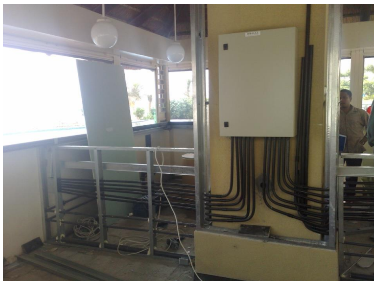
ELECTRICAL WORKS @ IFA CLUBHOUSE-PALM JUMEIRAH
