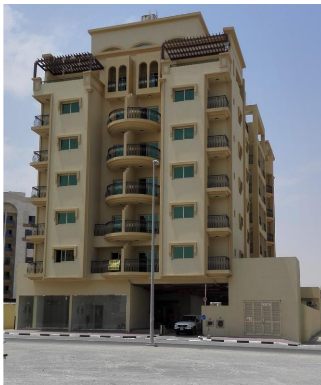
B+G+6+GYM+ROOF BUILDING @ AL WARQA 1
