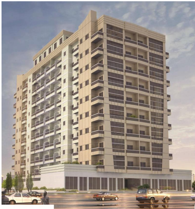
ELECTRICAL WORKS @ 2B+G+9 BUILDING @ MUHAISANAH FOURTH
