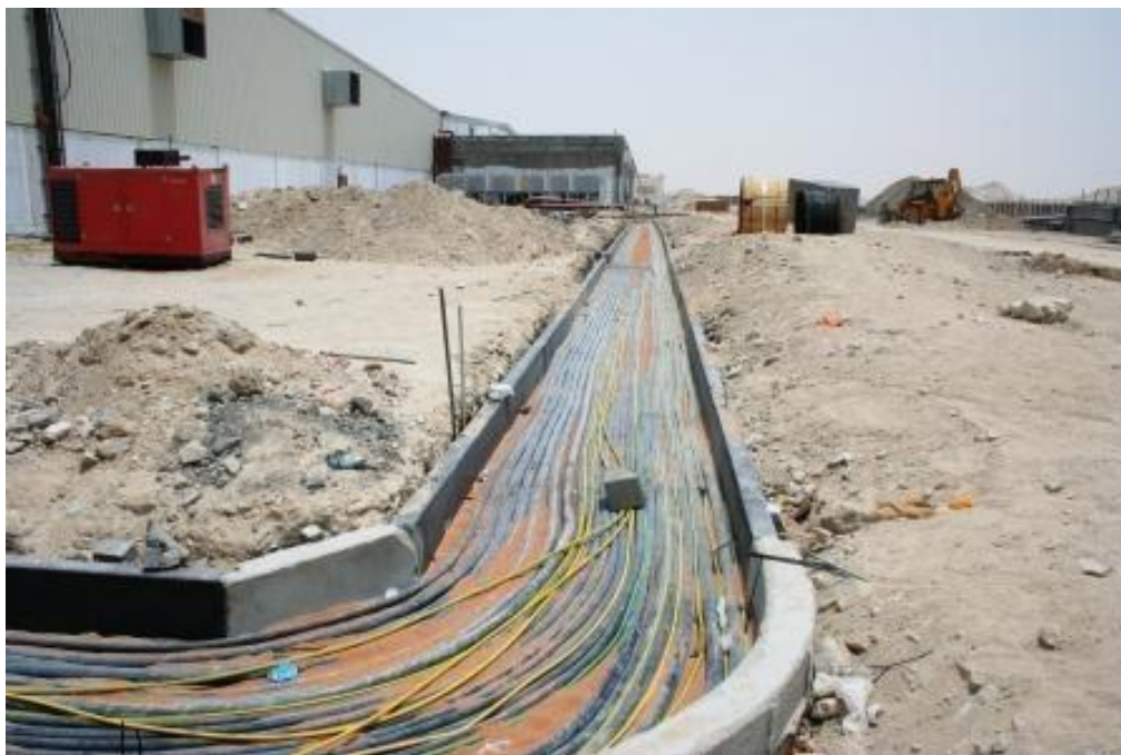
CABLE LAYING WORKS FOR INTERNATIONAL CAP @ JAFZA
